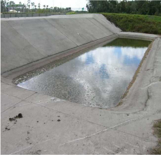
Drainage Outfall at Mainline Barrier Plaza
